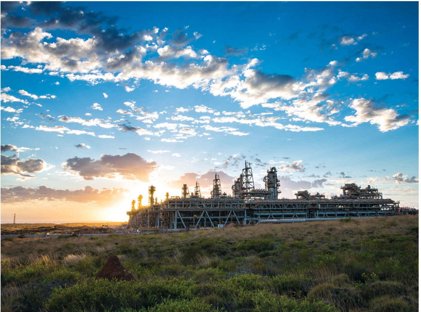
Startup of the third LNG train at the Gorgon Project was achieved in March 2017.
